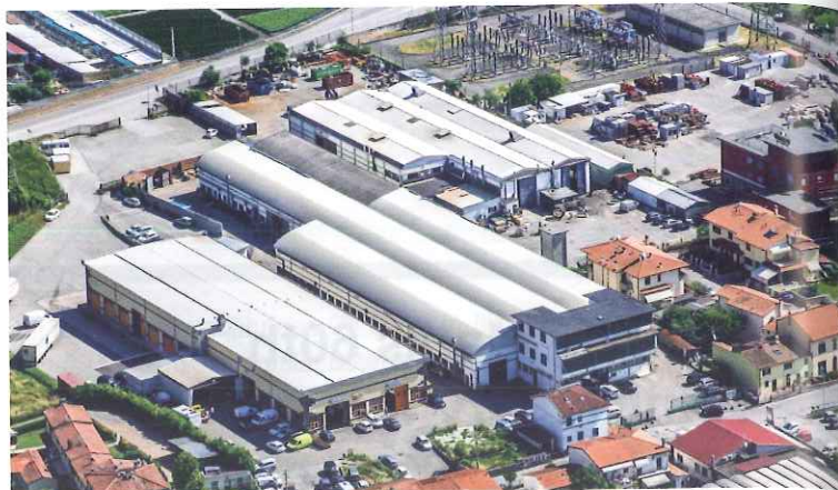
Cima's production facility, which recently benefitted from an investment of more than €800,000, manufactures equipment designed by the company itself
